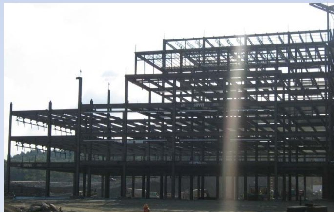
East Building Steel
