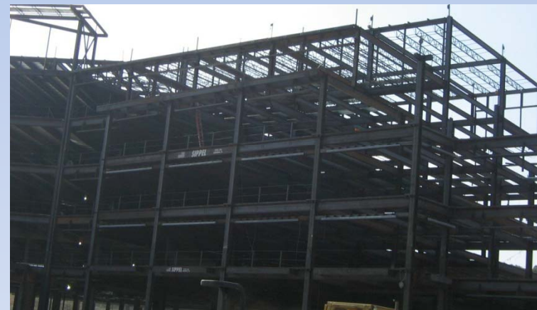
West Building Steel
